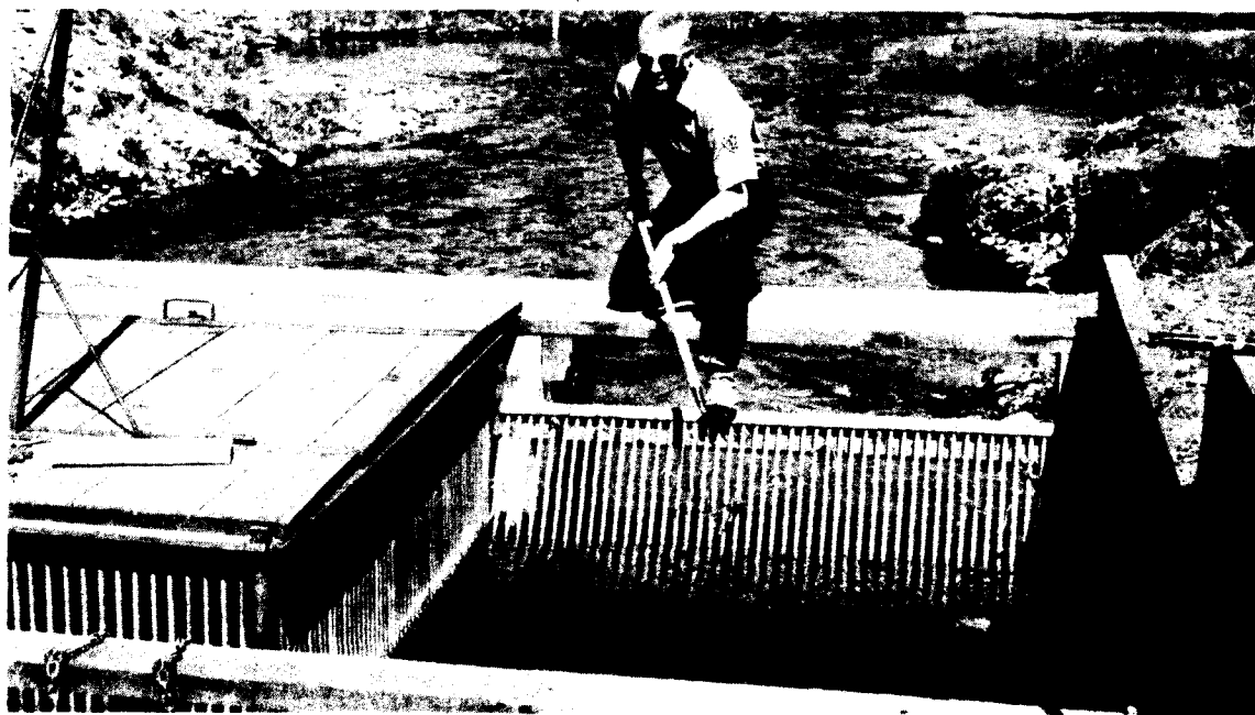
Fish weir used to count salmon and steelhead entering and leaving the upper portion of the Lemhi River.
